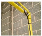
Run the trace heating cable along the inlet pipe and turn through 90 degrees vertically up the pipe to the top shower valve, the electrical cable should be looped around the valve as shown and secured using tie wraps or PVC tape (not included)
