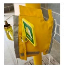
Cover #4 fits around the eyewash valve and inlet pipework it has two holes in the cover, it should be positioned as the image on the left, to ensure correct orientation around the eyebath valve.
