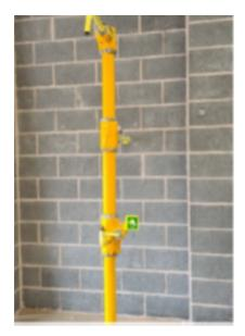
Install the 3 pre-assembled straight lengths of yellow foam insulation using the Velcro fastenings onto the straight large diameter upright pipe lengths, as shown.
