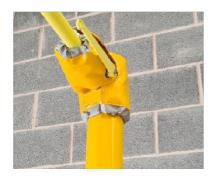
Starting from the top, fit the valve cover #1 onto the shower valve securing with the Velcro flaps & side drawcords. Cover #2 will fit over the Tee section at the top adjacent to cover #1. Ensure the upright foam lagging is inside the drawcords joint before tying securely.
